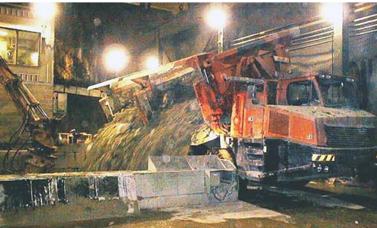
Henderson Mine ore truck discharging ore into the crusher.
