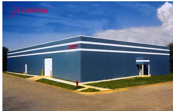
Load Cell Production Building
